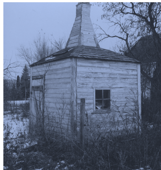
Figure 58 Wood frame smoke house located on the P. Suderman farmstead, Village of Neuenburg.
