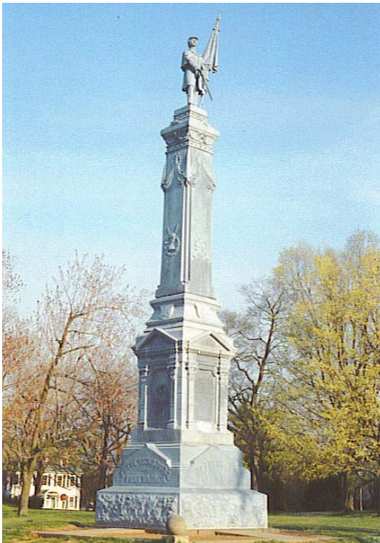
Civil War Memorial in Stratford, Connecticut, 1889. Like this one, a number of Civil War memorials are constructed of cast zinc (or “white bronze”), a process that became available in the 1870s. Relatively inexpensive, it enabled communities to erect very large and ornate monuments like this one, which lists the names of those who died. (Jon Best)
